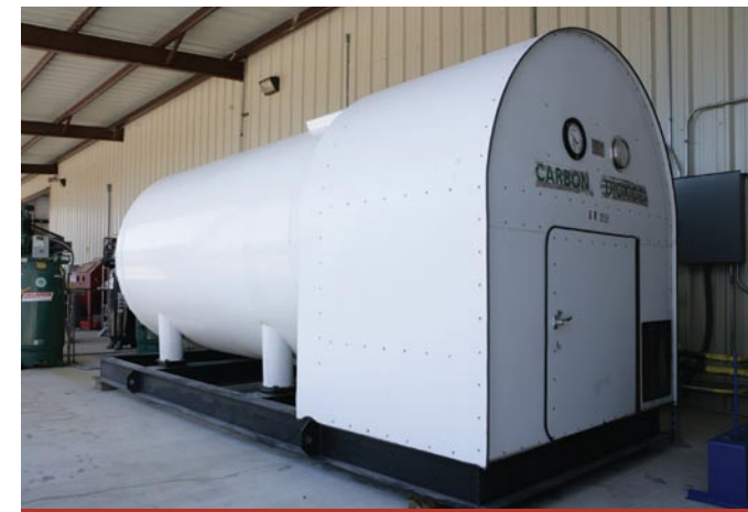
BULK CO 2 TANK
